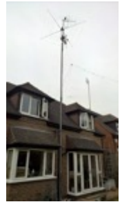
Medium size antenna 160m-6m (HF-Shortwave radio)
